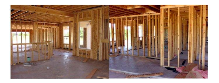
The first phase of construction includes lot clearing, setting foundation forms, roughing in the plumbing, digging beams, placing steel, and finally pouring the slab. Soon after the slab is poured, framing begins and you will be able to experience your new home three dimensionally for the first time.
