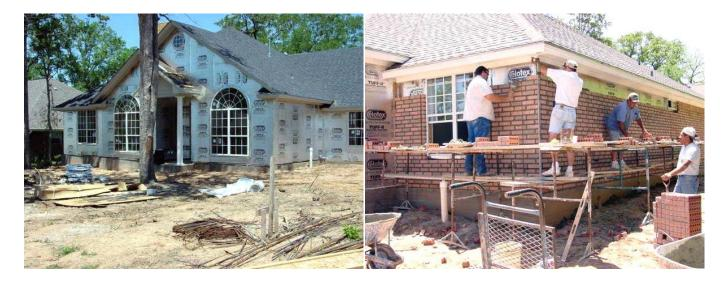
The activity continues with wiring, topping out the plumbing, roughing in the mechanical, and measuring for cabinetry. Meanwhile, the outside of your house is being "dried in" with primer paint, roofing, and masonry.
