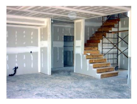
Once the drywall is in place, the walls are textured, and work begins on trimming and setting the cabinetry. During these phases of construction, we work with you to select colors and finishes.
